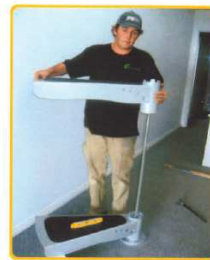
(4) Bolt allthread to bottom tread which has three grub screws inserted, then place over base plate. Pack under end of tread to level. Tighten up grub screws.
