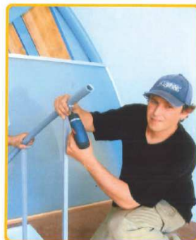
(8) Screw fix handrail to main balusters.
