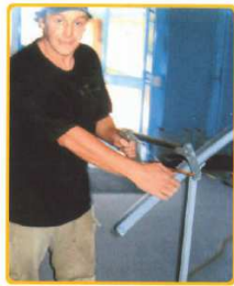
(10) Cut handrail to length then fit end caps top and bottom.
