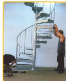
(9) Add middle balusters to stair. Again using centre column as plumb guide. Screw fix balusters to handrail. Leave off front baluster to floor and top baluster to landing
