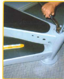
(6) Tighten down centre column nut on all treads as you install them after main baluster is bolted tight.
