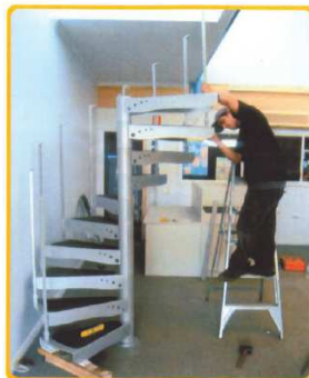
(7) Bolt all treads and main balusters on stair then connect top riser pipe to landing.
