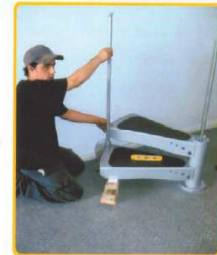
(5) Bolt main baluster post to tread. Align by eye with centre column for plumb, and tighten bolts on baluster.
